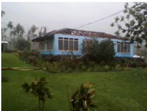
house with roof blown off.jpg 39K
