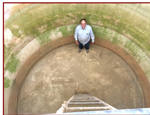
16,000 gallon underground tank
