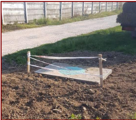
Underground water meter
